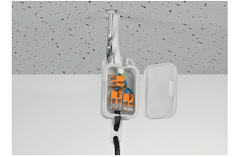
Pendant light connection in a suspended ceiling
