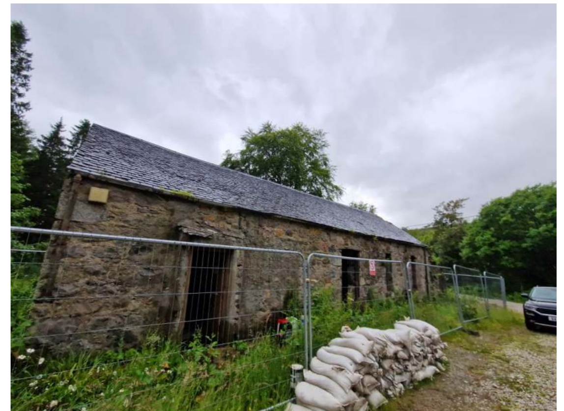
Fig. 8 – The north elevation of the subject building.
