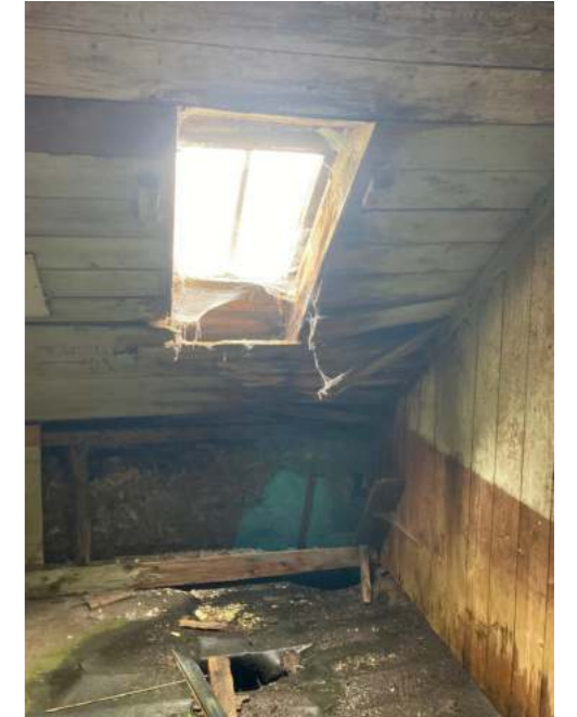
EXISTING ROOF LIGHT
