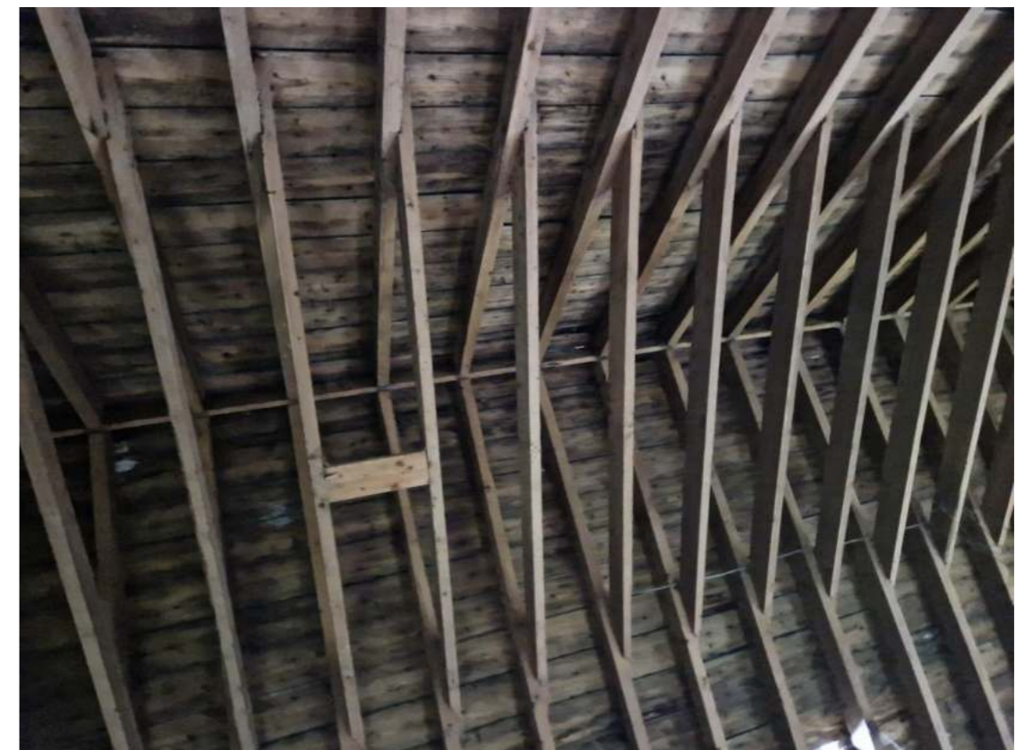
Fig. 16 – An example of the interior roof structure.
