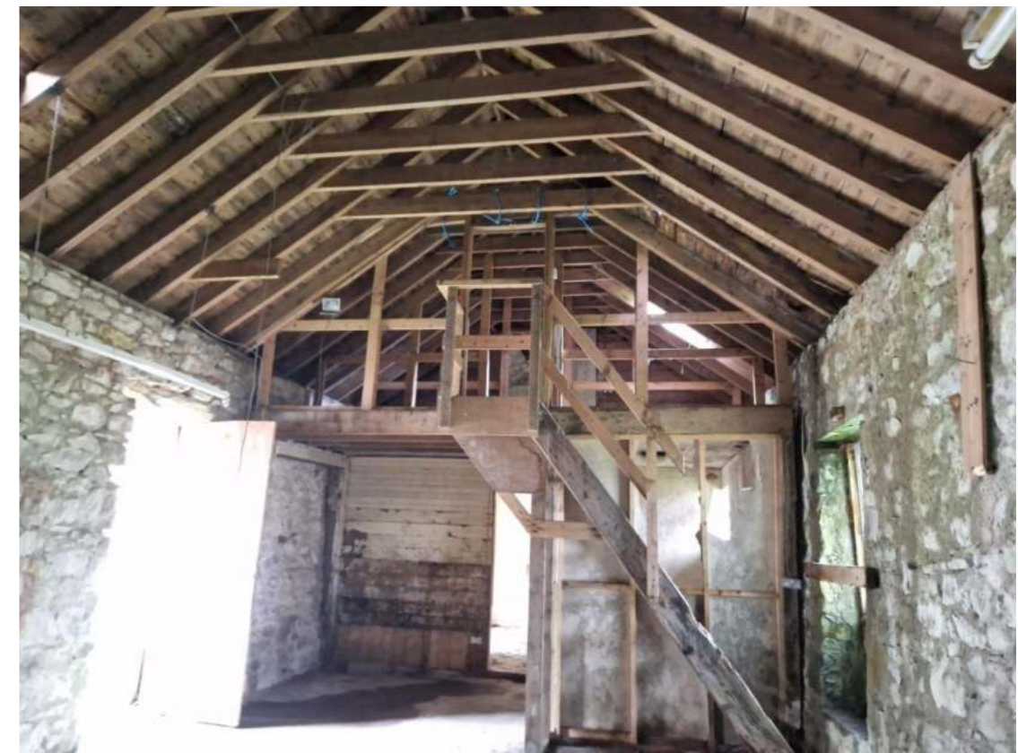
Fig. 15 – An example of the interior structure of the subject building.
