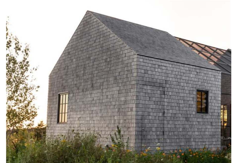
TIMBER SHINGLES Used to create texture and reflect traditional techniques. (Berman Horn Studio)
