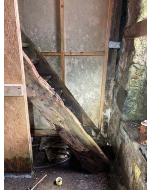
EXISTING STAIR ACCESS
