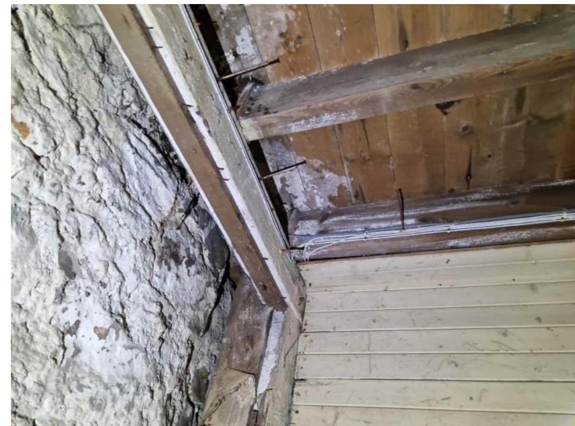
Fig. 12 – Example of the sarking and roof joists.
