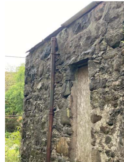
BLOCKED UP WINDOW OPENING
