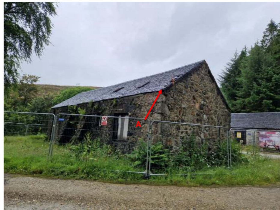
Fig. 22 – The south and west elevations of the building, denoting roost A.
