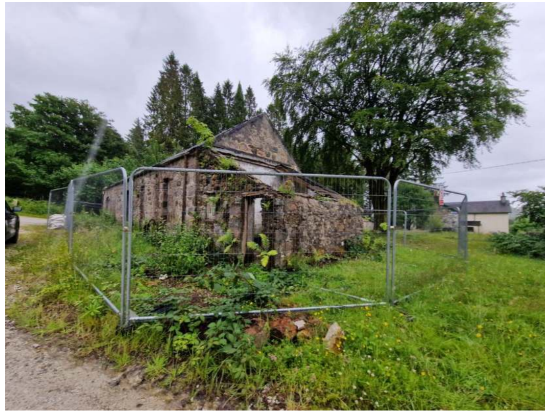
Fig. 9 – The north and west elevations of the subject building.
