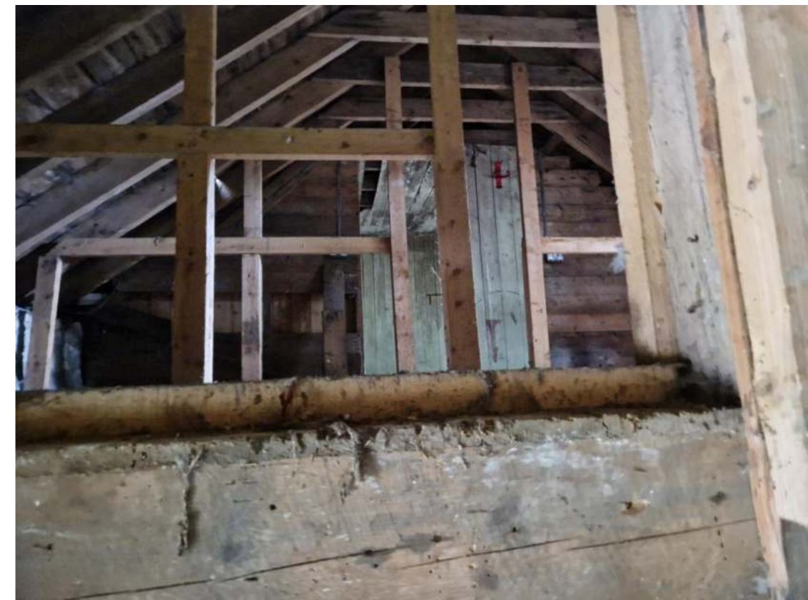
Fig. 11 – The upper storey as seen from the staircase.
