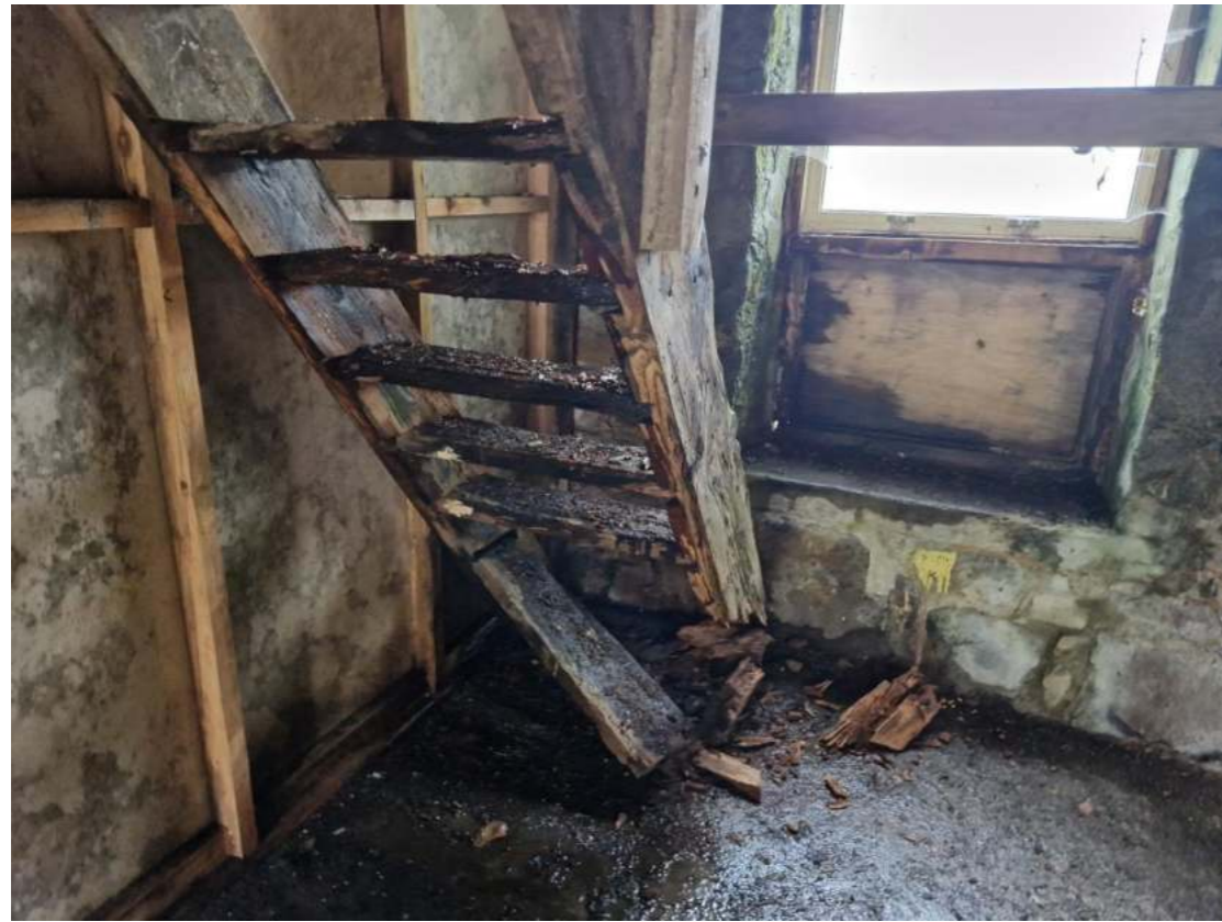
Fig. 17 – The inaccessible staircase.
