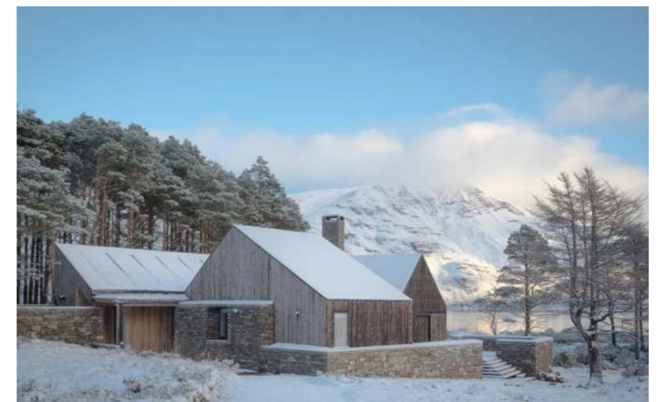
LOCHSIDE HOUSE - HAYSOM WARD MILLER
