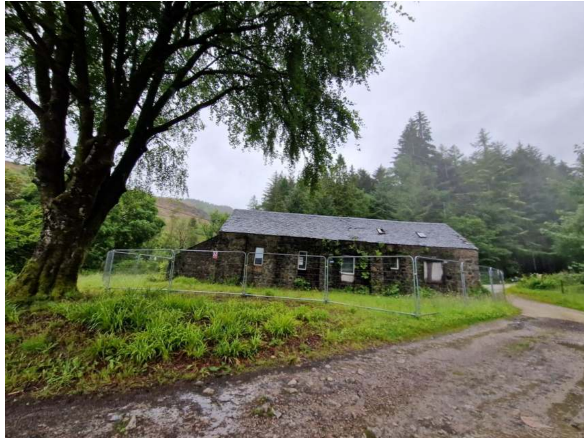
Fig. 6 – The south elevation of the subject building.
