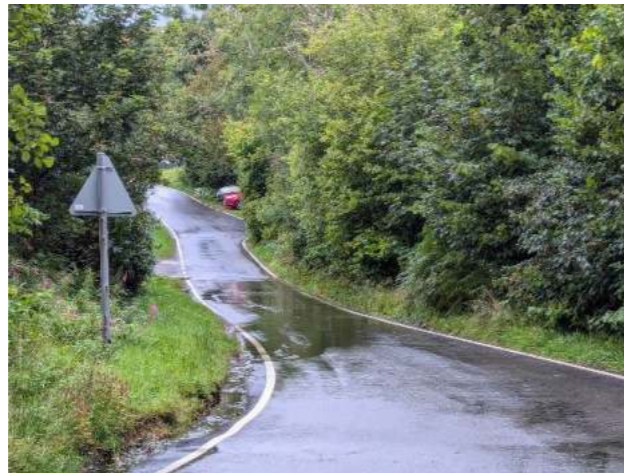
Figure 3 - Passing Places on access road
