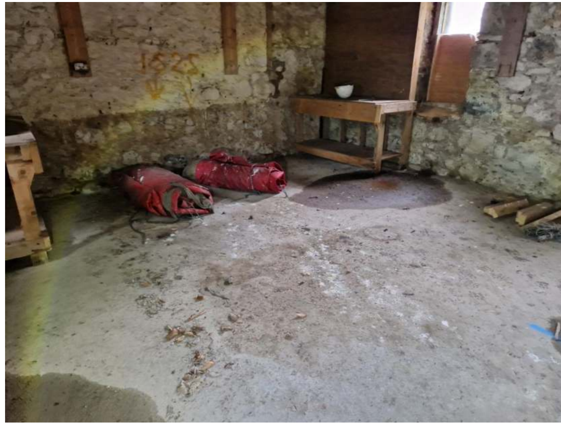
Fig. 13 – The interior of the subject building.
