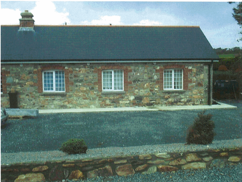
Renovated gate lodge
