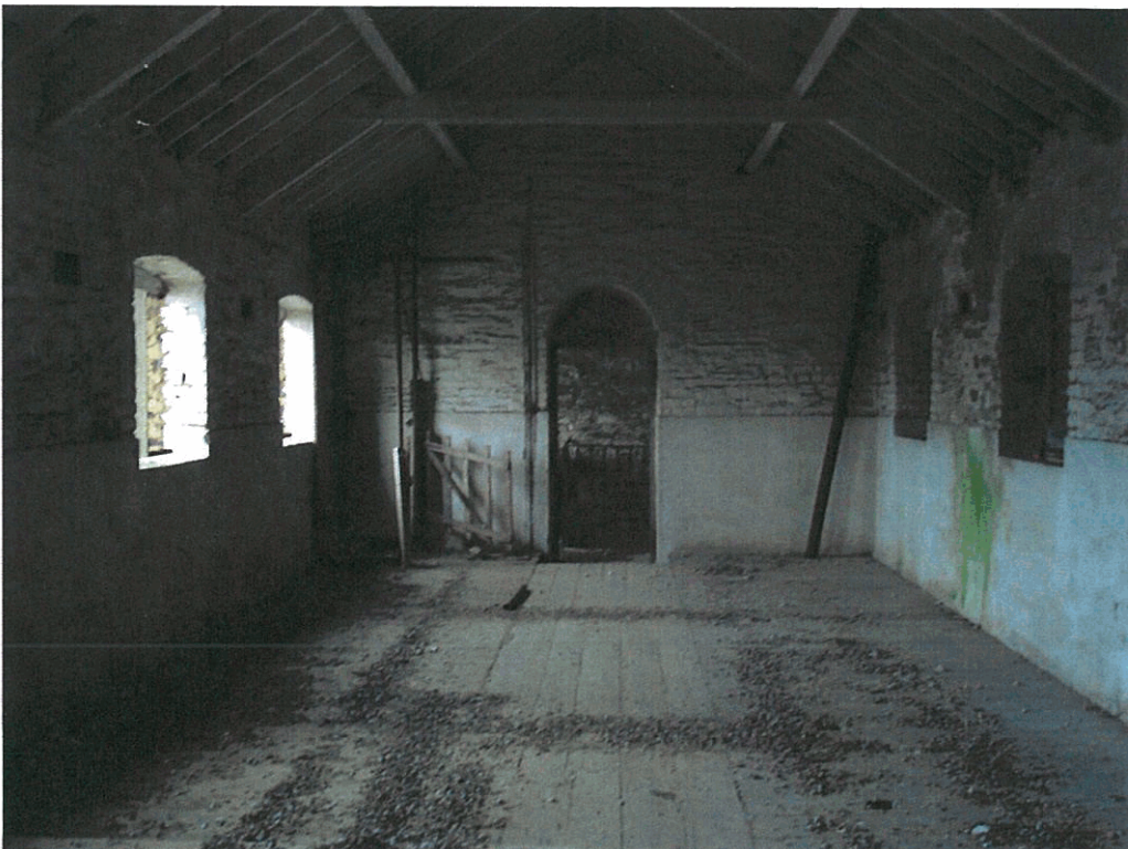
View towards the stairway from the upper female dormitory.
