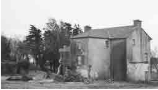
Pictured Above is Ballinacourty House in 1900
