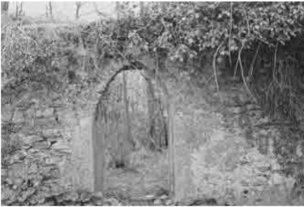
Pictured above are The remains of the Walled Garden in Ballinacourty in 1900s
