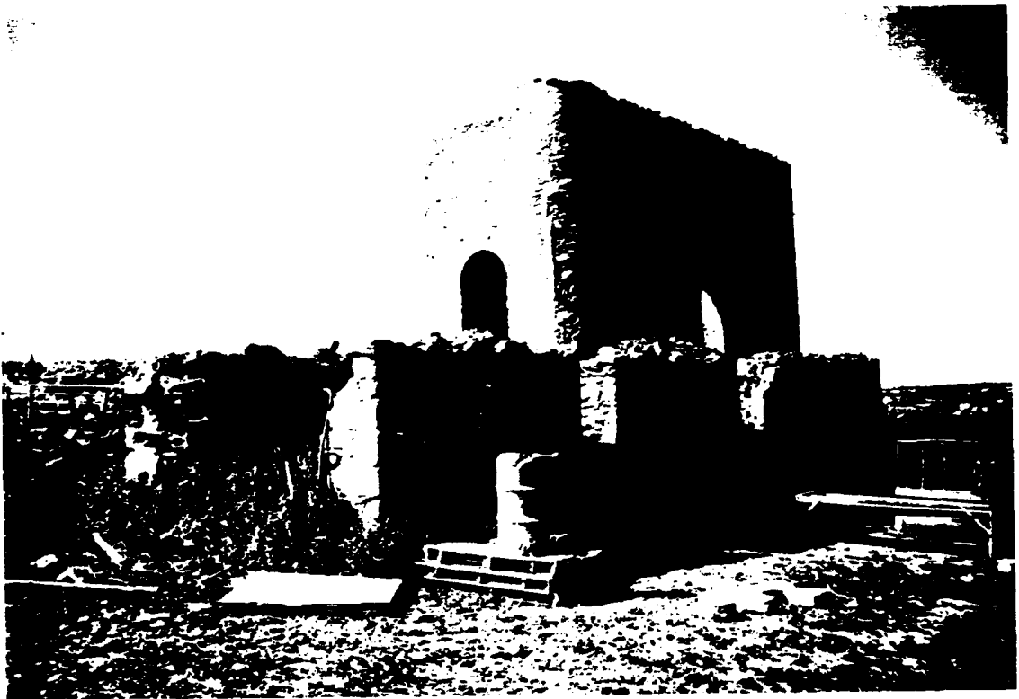
Fig 7. This engine house was probably built in the 1860s to pump the Tankardstown mine as it extended northwards
