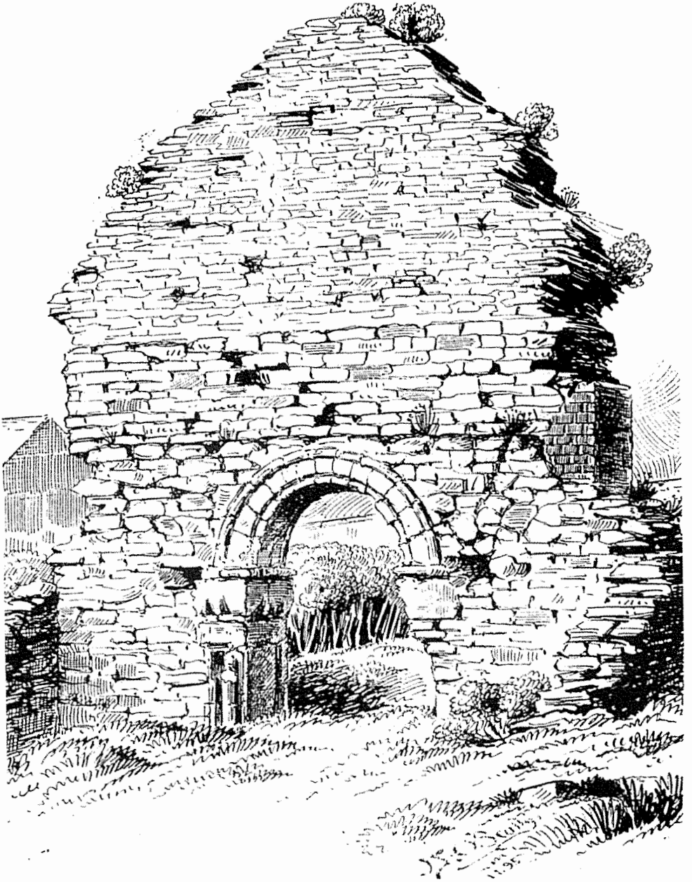
St. Thomas' church, Thomas Hill Waterford, prior to its demolition in the 1960s.
