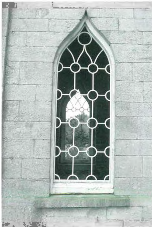
Figure 6: South facing window.
