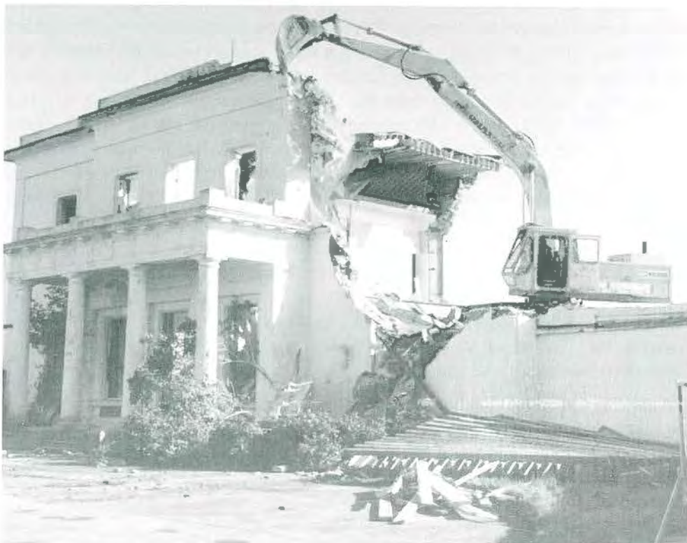
Figure 10: Demolition of Ardkeen House, 18 April 1988.
