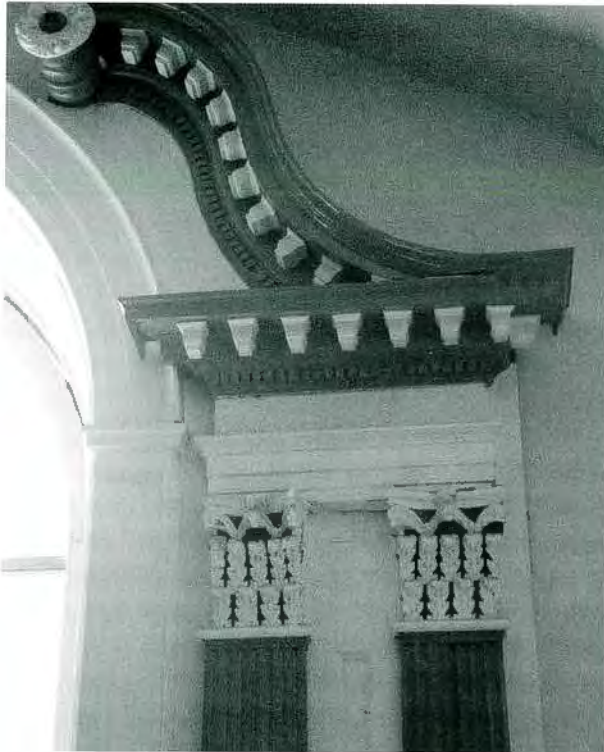
Figure 7: View of the United Methodist Presbyterian Church, Waterford, showing a section of the decorative frieze and cornice of the south window.
