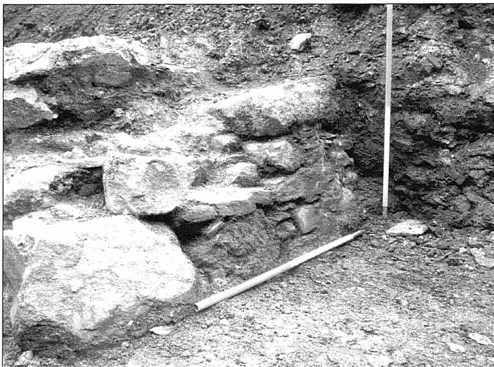
Plate 7 – Revetting wall from south-west.
