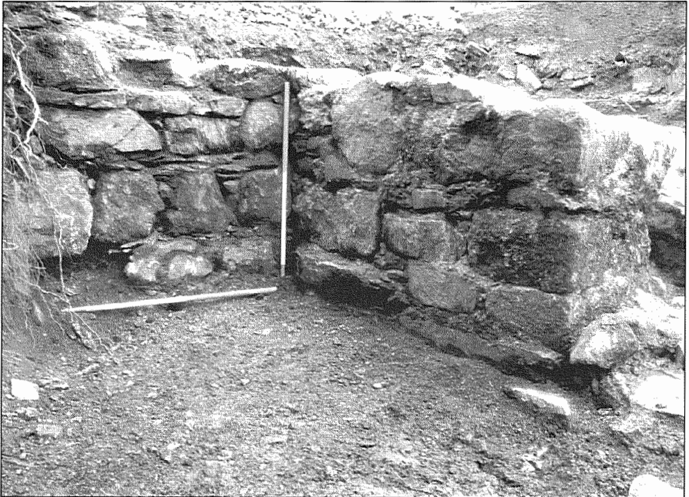
Plate 4 – Exposed masonry of city wall / Colbeck Gate.
