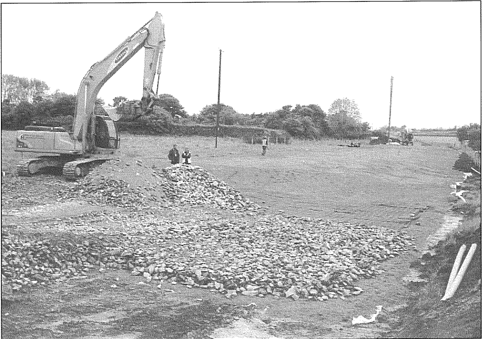
Plate 5 - Geogrid covered with hardcore material at 1180m.ch. and general view of site from south (02_50_CP16_13).
