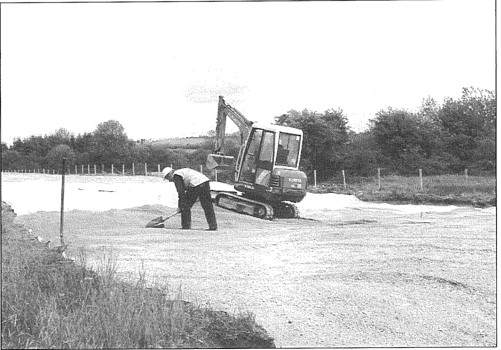
Plate 4 - Crushed stone spread over basal terram, 1160.m.ch. (02_50_CP16_20).
