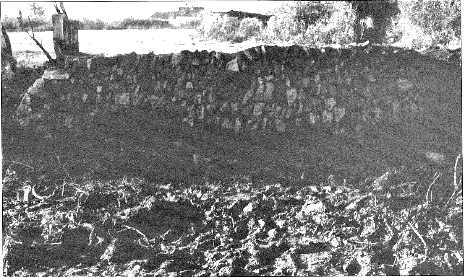
Plate 3 - Earthen bank with stone facing from east (02_50_CP7_16).
