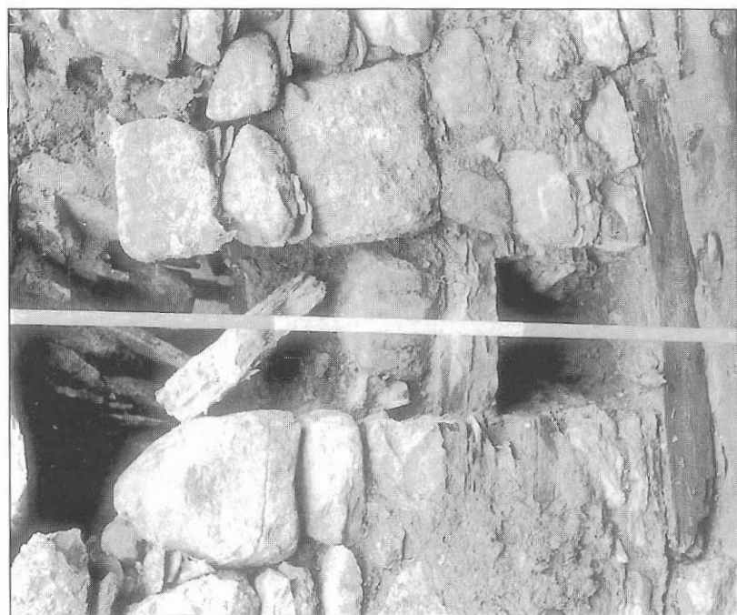
Plate 15 – Seventeenth century sluice exposed in Trench A that controlled the flow of tidal water in and out of the tanning vats within the Watergate – inserted into the sixteenth century blocked N-E archway (Arch D) of the latter. B.M. 1987
