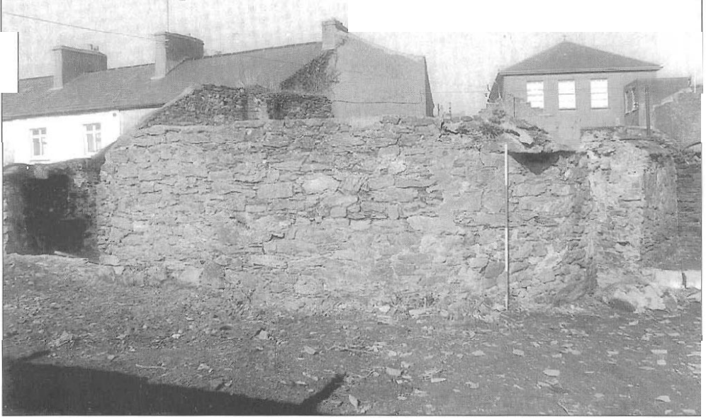
Plate 1 – The upper exterior of the Watergate from N-E, prior to the commencement of excavations in Bergin's Garden in 1985.
