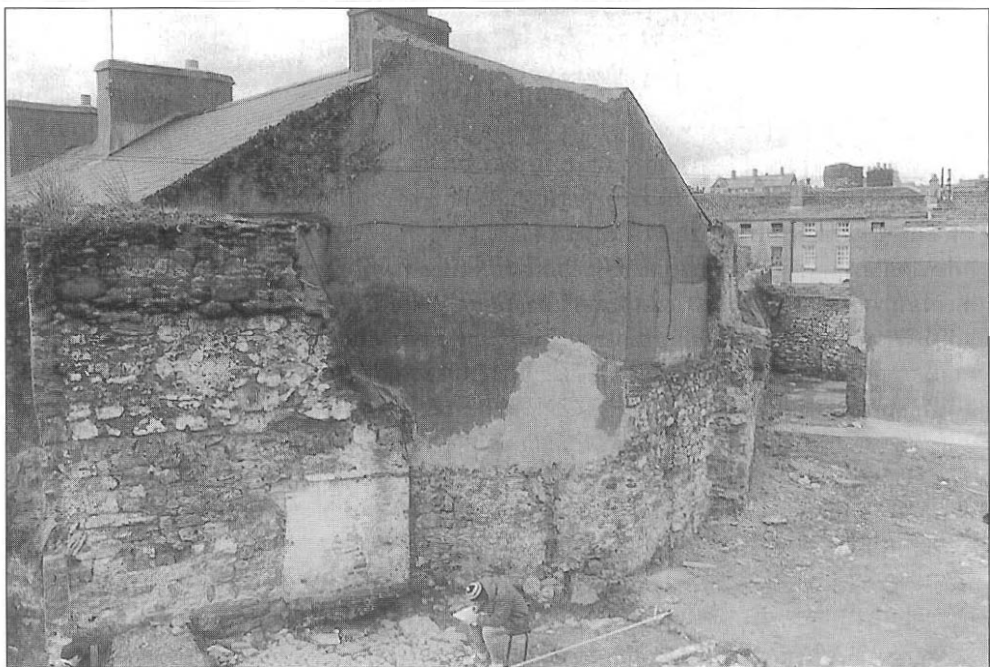
Plate 5 – View of N-E end of late Georgian terraced houses fronting onto Mendicity Lane from Grady's Yard, during the first season of excavations in 1985 – showing the wall-walk level of the inner face of the Watergate, on the left and the end of the city wall above ground level on the right.
